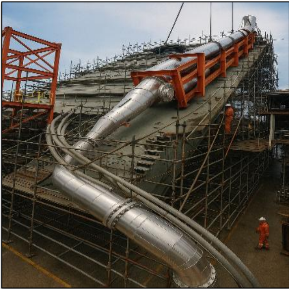
SEP-iSYS™ for TGT FPSO in Vietnam 2011
